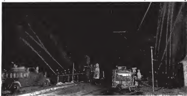
Twelve streams of water flow as two pumps build up pressure.
